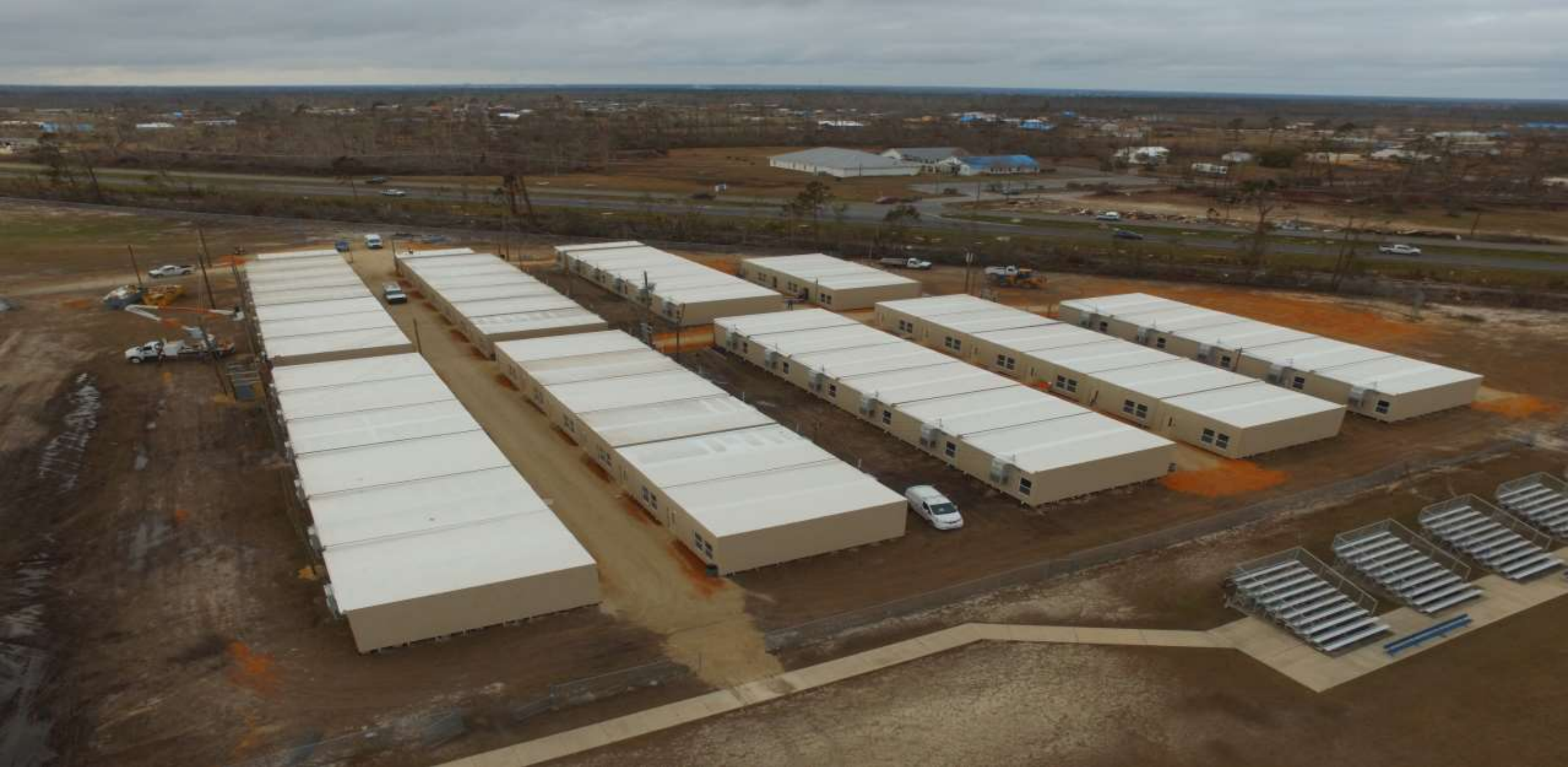
Modular units set up to house students as of January 22
