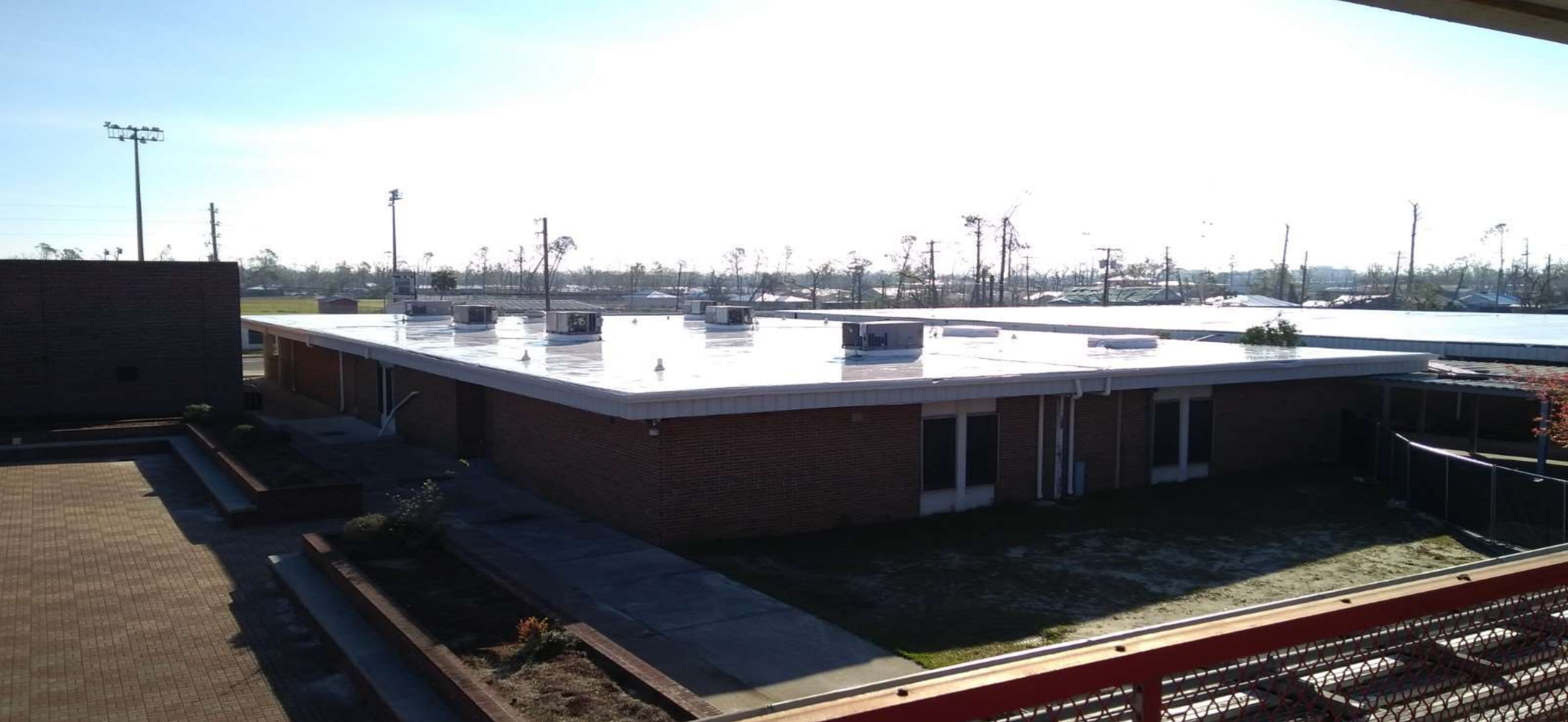
TEMPORARY ROOF REPAIRS BEING AT MADE BAY HIGH SCHOOL
