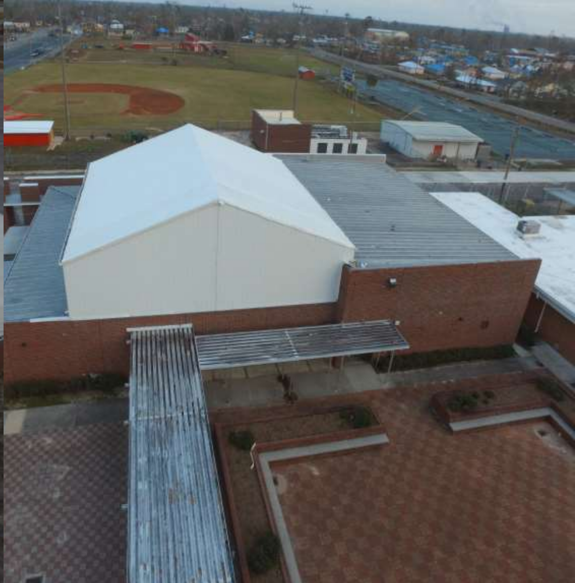
BAY HIGH BANDROOM ROOF AND THE TEMPORARY ROOF REPAIR
